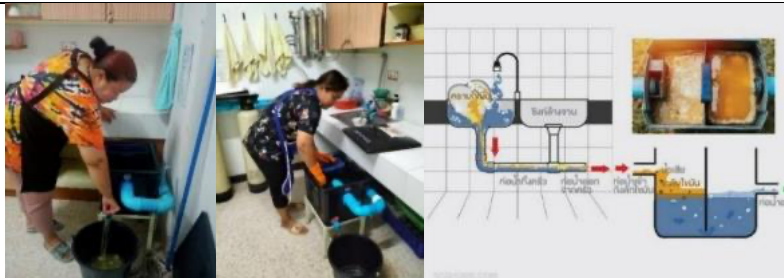
Picture the installation of a grease trap.
