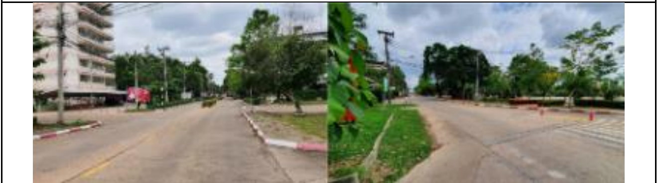
Image of the traffic routes inside the university
