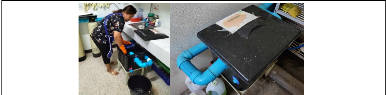
Installation of ready-made treatment tanks
